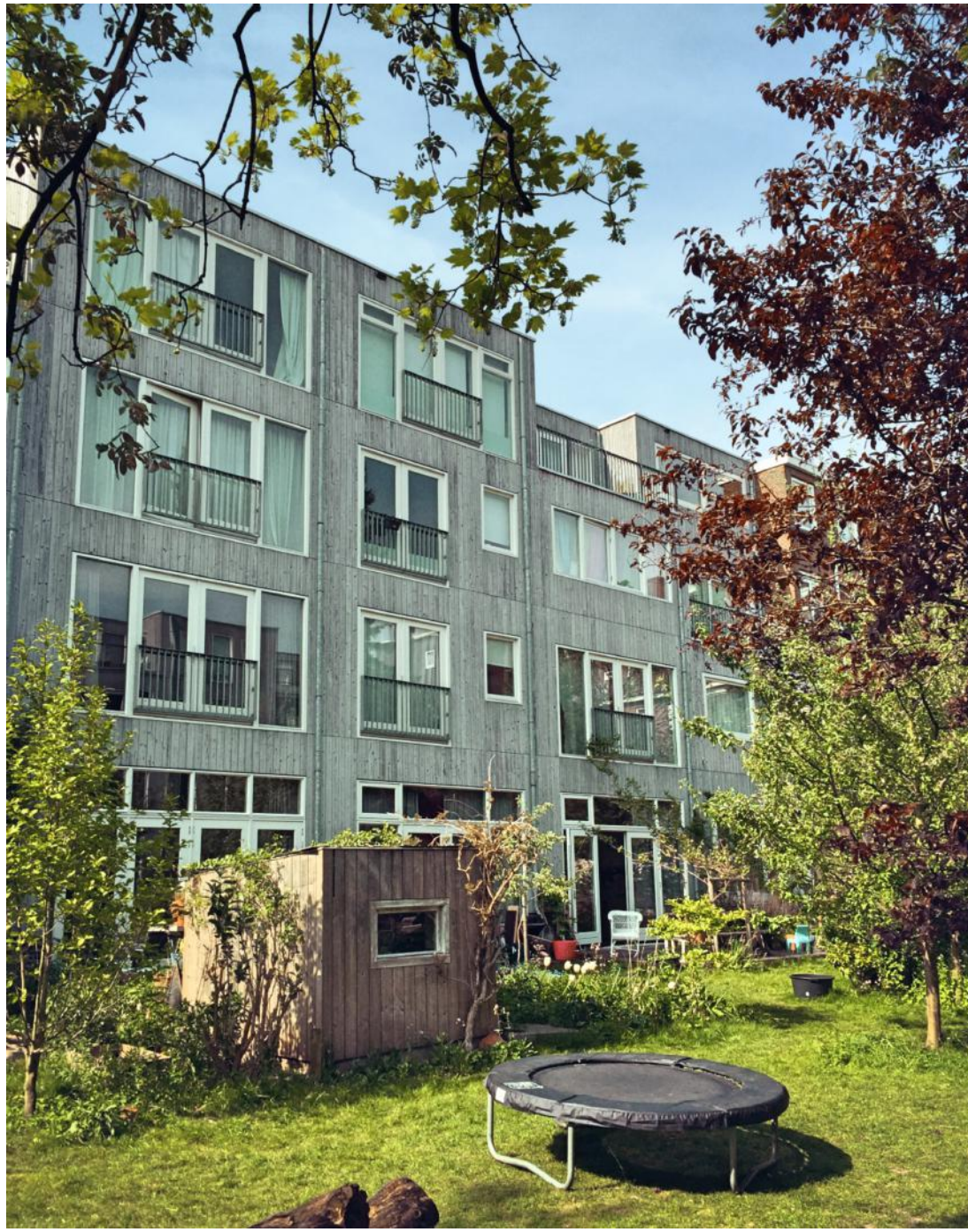
Walisblok, Rotterdam, fot. At
